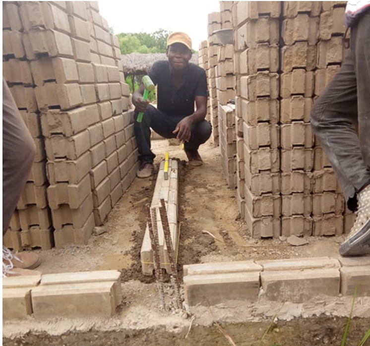
The mason laying the first course of bricks
